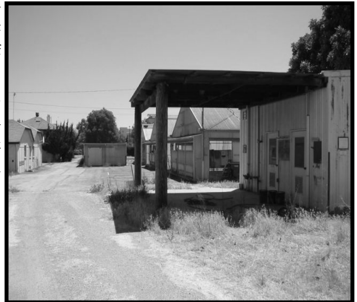
BAREC – Looking east, shop on left side, potting shed, greenhouses and chemical shed to right.
